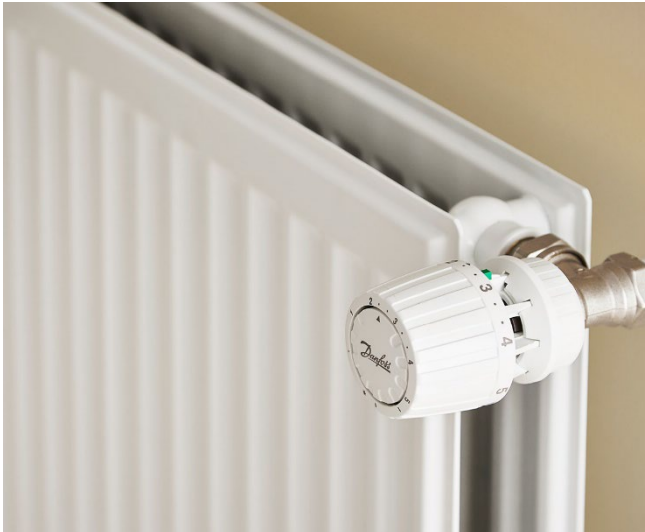
Figur 18: Panelradiator - type PII
