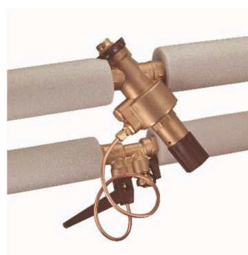
Figur 11. Dynamisk ventil (trykdifferensregulator)
